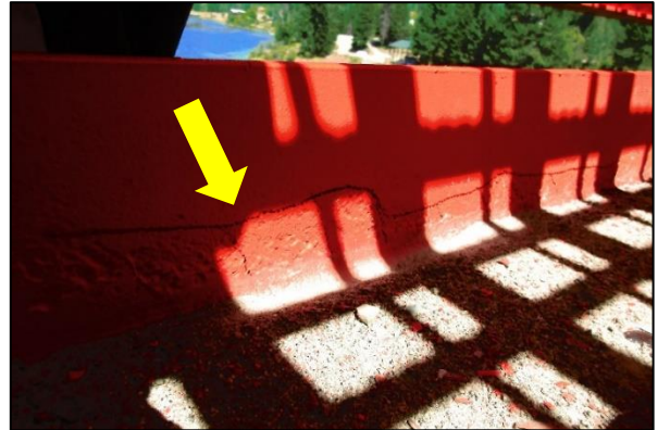
Photo 12. - Pitting corrosion in top chord where debris can build up.
