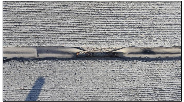
Photo 10 – Failed Deck Joint
