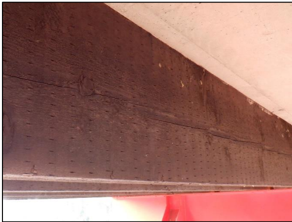
Photo 7 – Heavy Checking in Girder 11H
