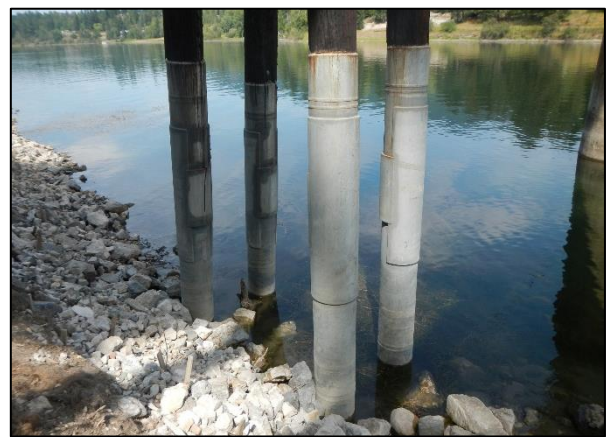
Photo 4 – Spliced timber piles at Pier 7
