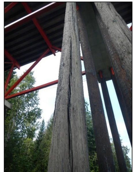
Photo 6 – Pile 7D up to 2-inch wide checks
