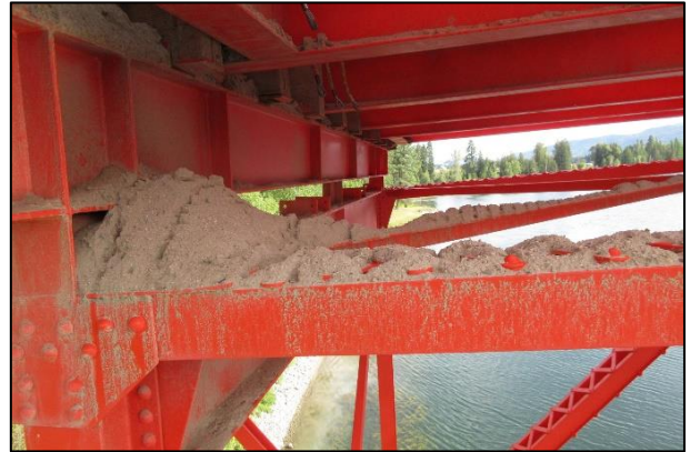
Photo 11 – Heavy debris accumulation at beginning of steel decking.
