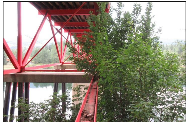
Photo 13 - Vegetation encroaching on truss
