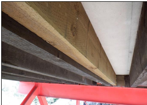
Photo 3 – Helper beam at Girder 13G
