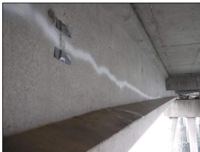
Photo 8 - Hairline cracking in girder web along path of harped strands.
