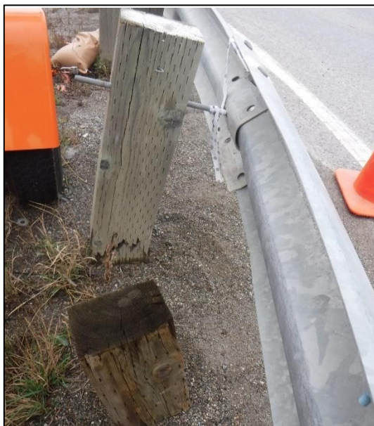
Photo 16 – Approach guardrail damage
