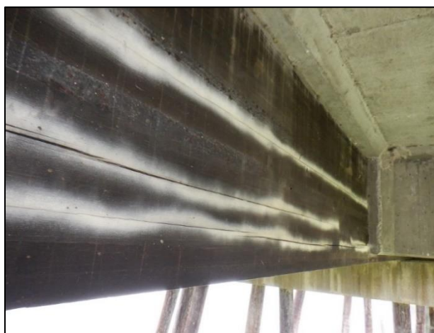
Photo 5 – Checking in glulam girders (highlighted in white)
