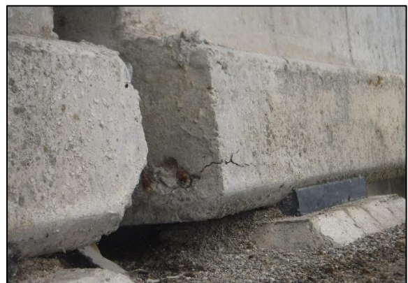
Photo 9 - Crack propagating at end of girder
