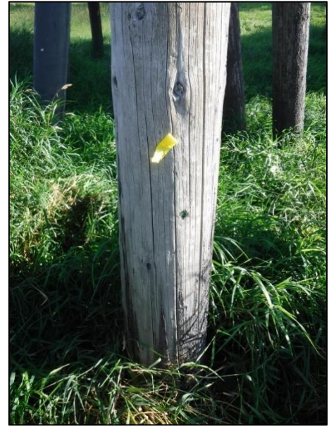
Photo 12: Yellow-tagged timber pile
