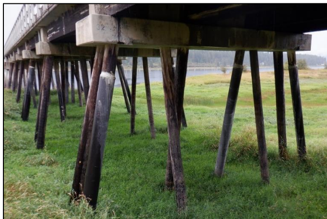
Photo 2 - Timber pile jacketing (Bent 32)
