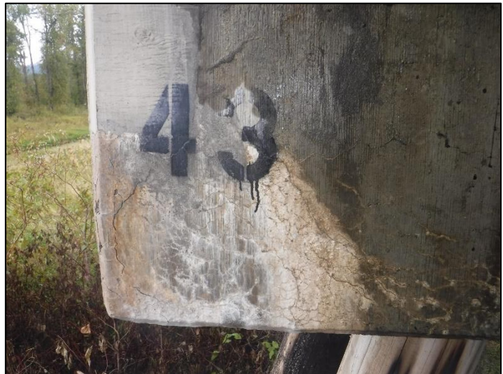
Photo 14: ASR Damage at bottom corner of pier cap.
