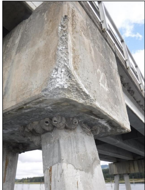
Photo 13 - Exfoliation at corner of pier cap
