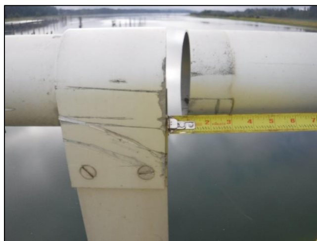
Photo 17 - Open gap at longitudinal bridge rail
