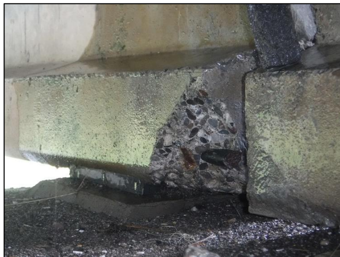
Photo 7 – Typical spalling at end of girder
