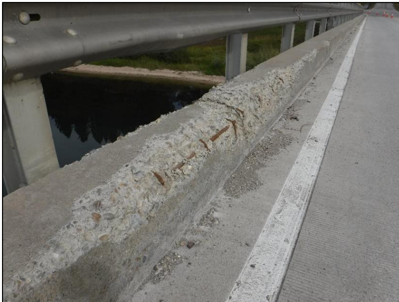
Photo 15 - Exfoliation of curb with exposed rebar
