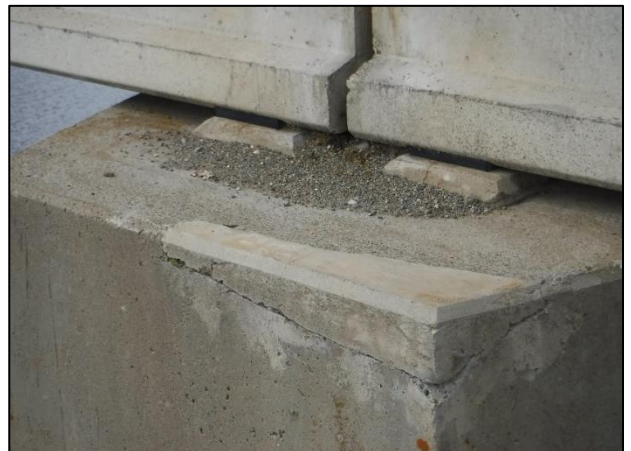
Photo 3 - Pier cap spalling repair
