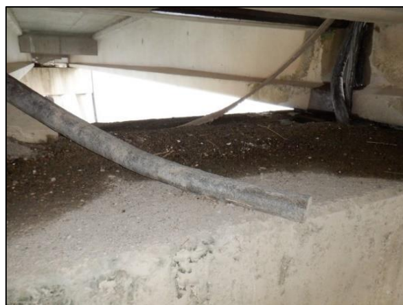
Photo 11 – Joint failure and debris buildup on pier cap
