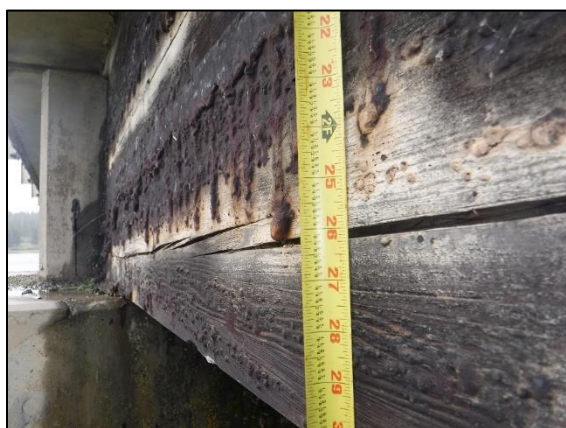
Photo 6 – Closeup of checking in glulam girders
