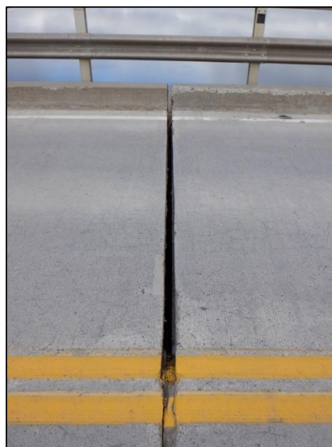
Photo 10 - Joint Failure showing open gap between girders
